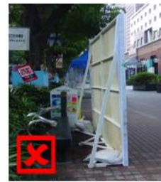
Exposed counterweight/ sandbags & brackets
