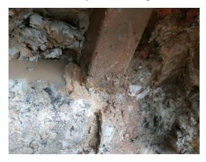
The incorrect construction sequence due to miscommunication on site resulted in the pile puncturing through a 'live' sewer.
