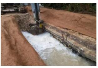
Tip of the excavator bucket punctured a water pipe at the construction site. This work was carried out within the vicinity of water pipe without approval from PUB.
