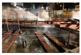
Necessary support structures not installed for the water pipe, as stipulated in the procedures for carrying out excavation work. This resulted in the water pipe being dislodged at its joint.
