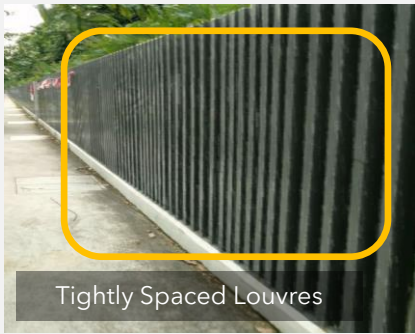
Figure 3.6 - Pedestrian access with Tightly Spaced Louvres
