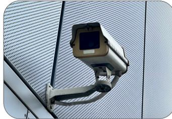
Figure 2: Bullet camera mounted on an exterior wall
