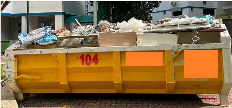
Figure 2 The side wall height of the OTC was extended using boards, grating and other materials.
