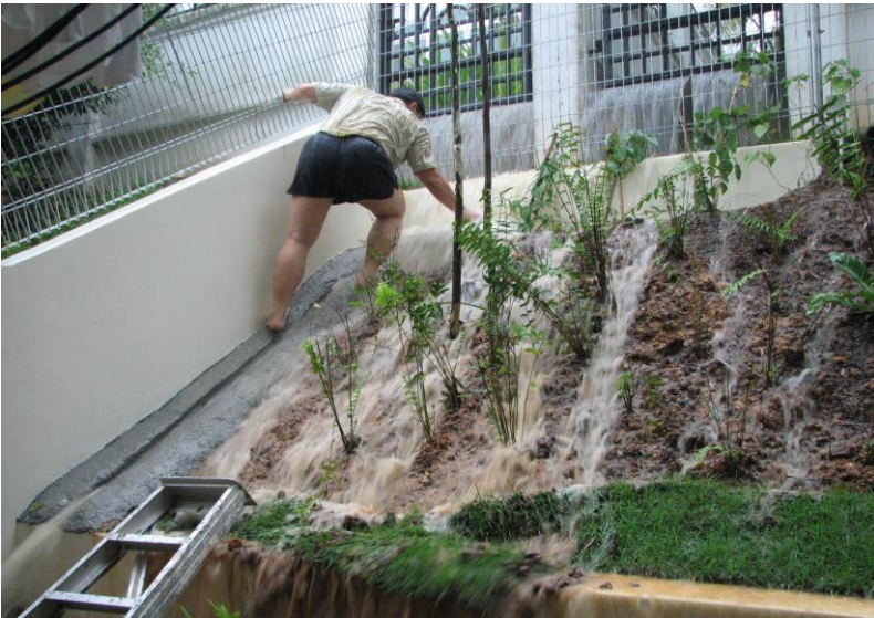
Water from development site on higher ground overflowing to the house at the lower ground
