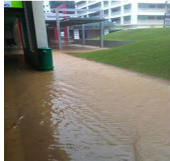
Surface runoff from higher ground flowing to lower ground area caused flooding as the perimeter drain is not sized for the additional catchment
