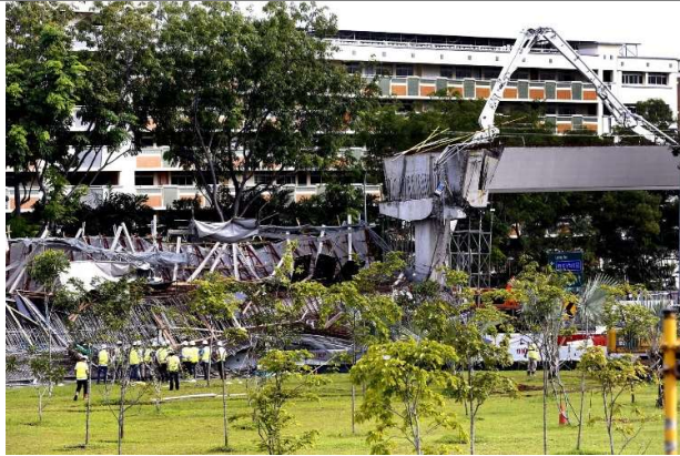
Collapse of bridge formwork during concrete pour
